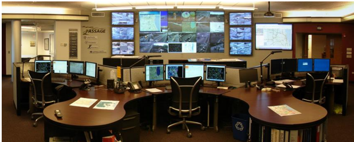
Figure 27: Lake County's Transportation Management Center in Libertyville
